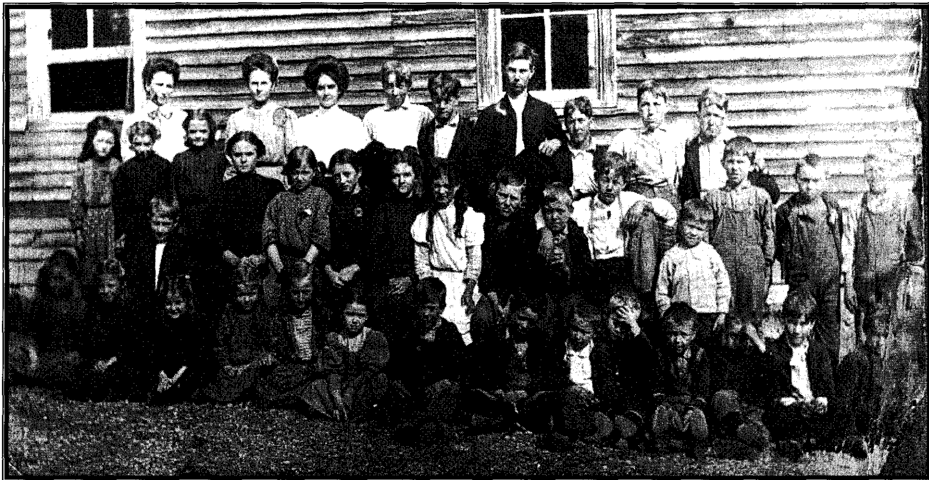
Figure 10.123. Salem Springs School. Photo was made about 1906.
